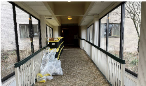
Ramp connecting various levels of the hotel
