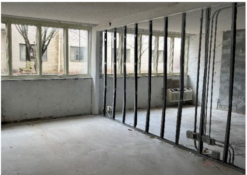
Hotel room demolished to the studs
